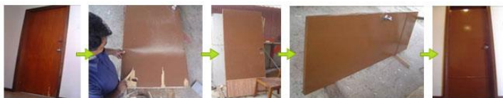
Image 20: Repairing a bathroom door (Frangipani Langkawi, 2014)
