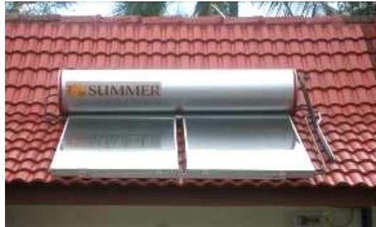
Image 19: Solar hot water system (Frangipani Langkawi, 2014)
